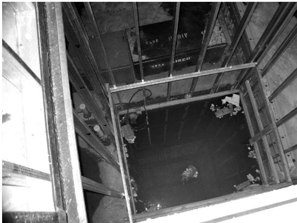
A view of the elevator shaft.
